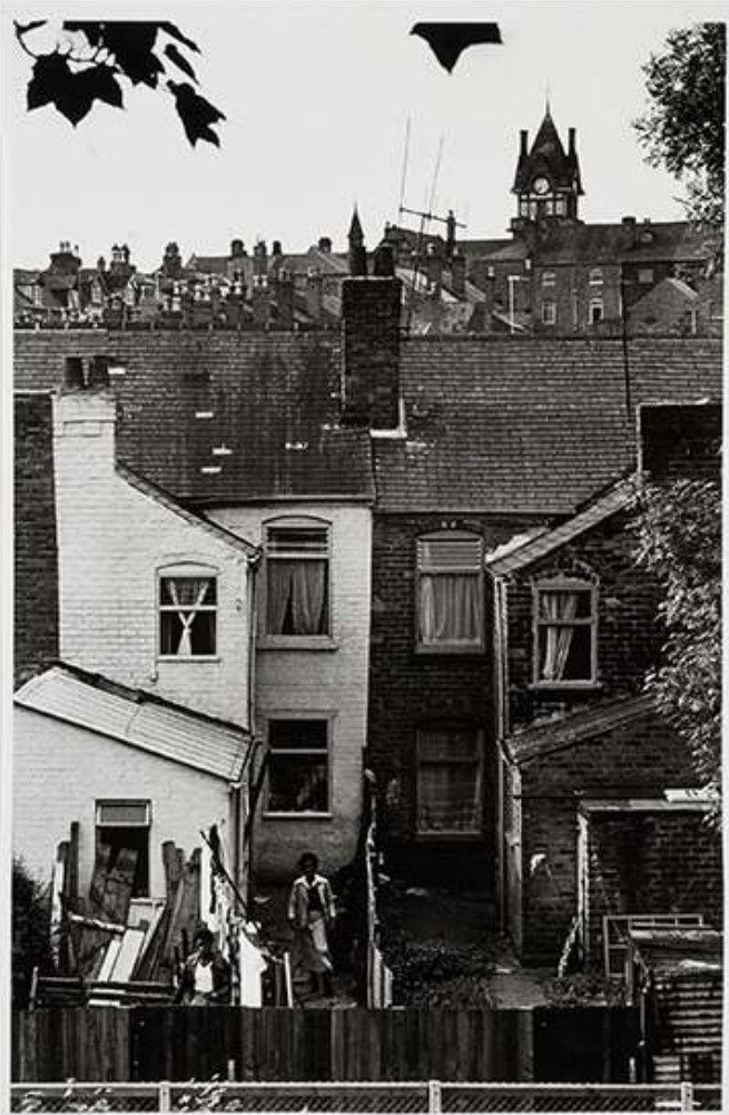
Vanley Burke, Back Garden from Railway Bridge , from the series Handsworth from Inside , 1968-1982. Arts Council Collection, Southbank Centre, London © the artist.
