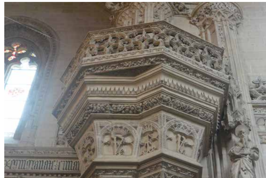
Fig. 8.18 Convent of San Juan de los Reyes, Toledo, detail of the decoration of the crossing piers, showing the initials of Ferdinand and Isabella (late fifteenth century).
