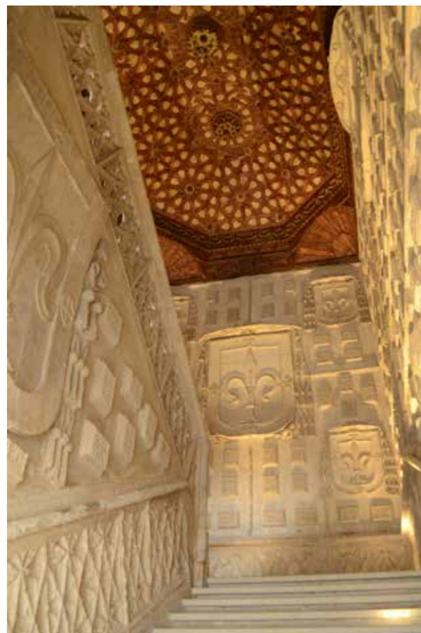
Fig. 7.14 College of San Gregorio, main staircase (1488–1496).
