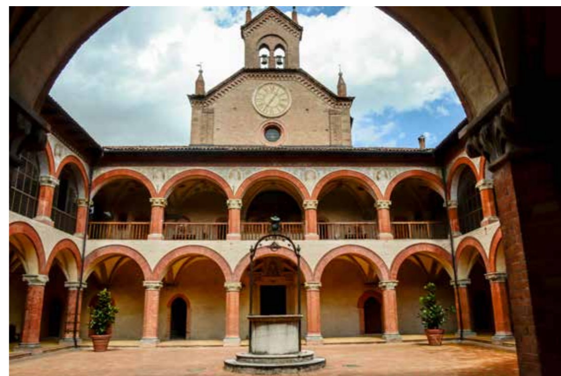
Fig. 7.2 College of San Clemente, Bologna (1367), main courtyard.
