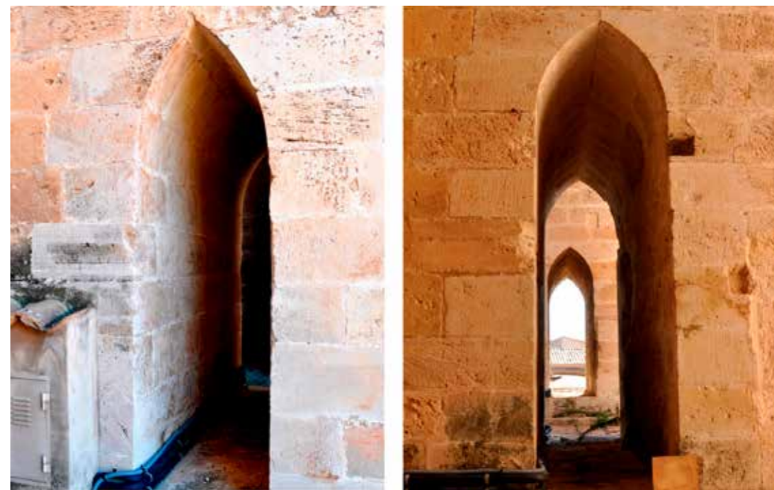
Fig. 3.14 Cathedral of Palma de Mallorca, passageways piercing the buttresses of the Royal Chapel (left: north; right: south) (early fourteenth century).
