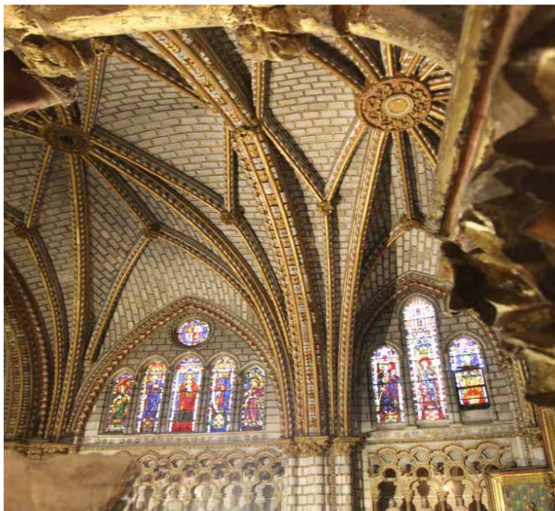
Fig. 1.12. Toledo Cathedral, presbytery vaults and triforium (ca. 1254–1274).
