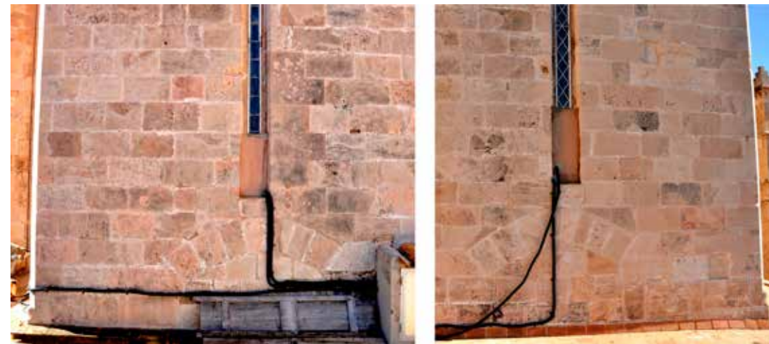
Fig. 3.8 Cathedral of Palma de Mallorca, discharging arches in the external sides of the Trinity Chapel (left: north; right: south) (early fourteenth century).
