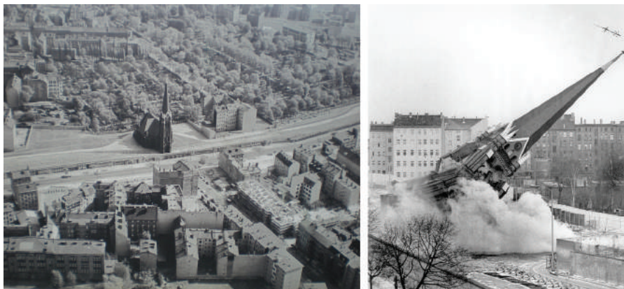
Figure 7. (a) The Reconciliation Church ( Versöhnungskirche ), Berlin, 1970; and (b) its demolition on 22 January 1985. Wikimedia Commons.
